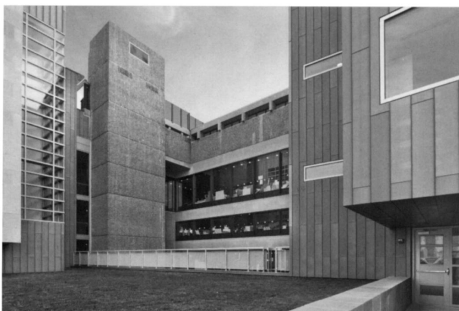
Fig. 7. Fourth-floor terrace and green roof, Paul Rudolph Hall, photograph 2008. Photograph by Peter Aaron, courtesy of Peter Aaron/Esto.
