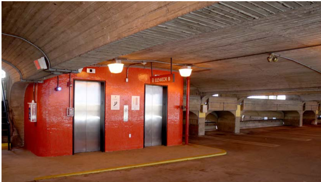
Photo 13. Interior view of upper level showing orange elevator bank, camera facing east. Note typical transverse structural beams overhead, and typical parking bays nosed in below structural bays at right.
