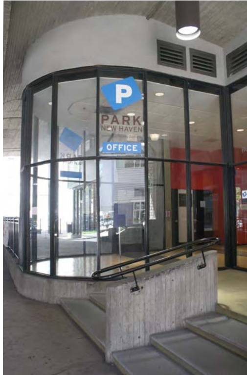
Photo 12. Exterior view of the George Street lobby (orange elevator bank), camera facing west.
