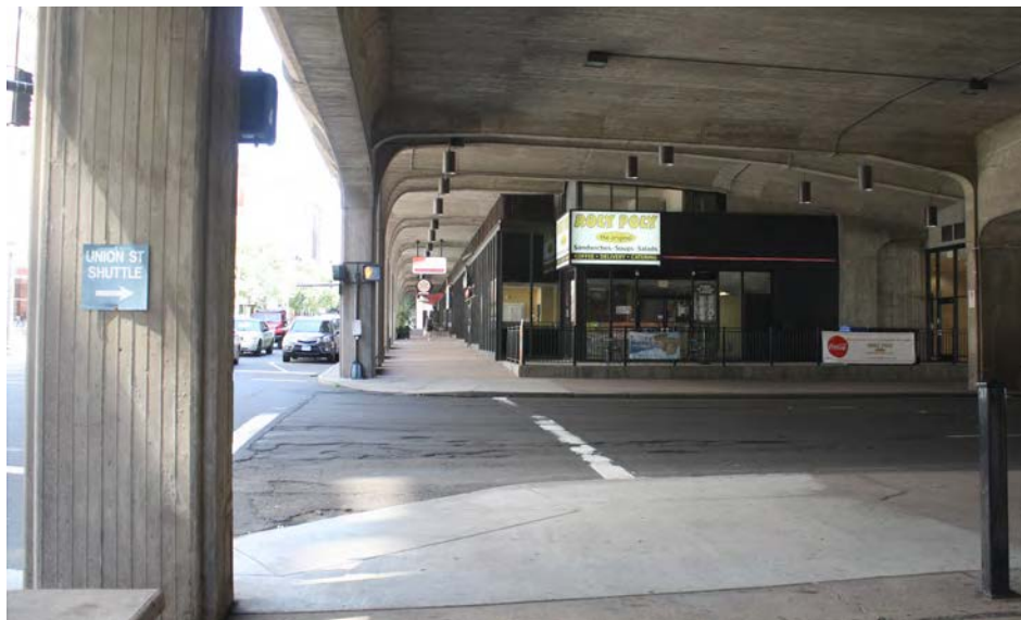
Photo 7. Sidewalk view along the west, Temple Street side of the garage, camera facing north. In the foreground is the intersection with George Street, and beyond the commercial space.
