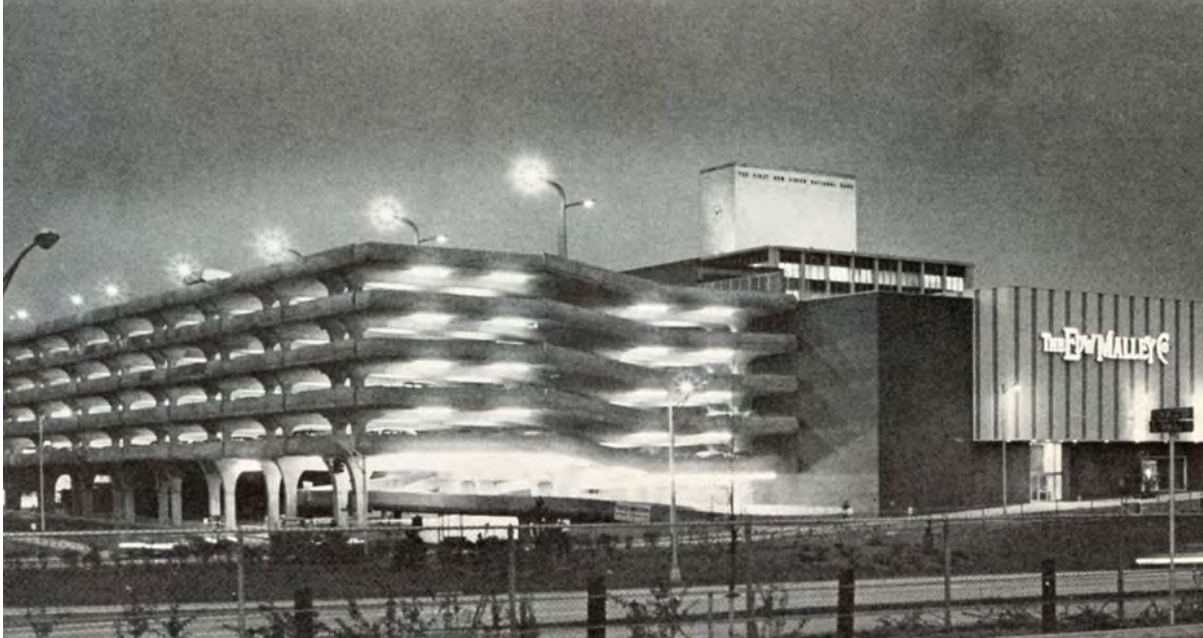
Figure 21. Southwest view of Temple Street Garage in the late 1960s; camera facing northeast, with the adjacent Edward Malley Co. department store. Photograph: New Haven Redevelopment collection, New Haven Museum.
