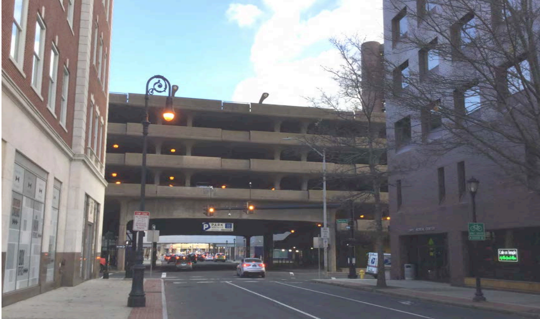
Photo 8. West view of garage at George Street, camera facing east, showing the garage spanning the street.
