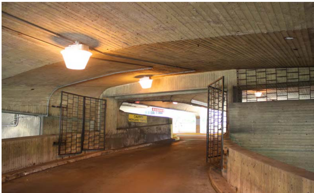
Photo 17. Interior view of ramp at south exit toward Frontage Road, camera facing south.
