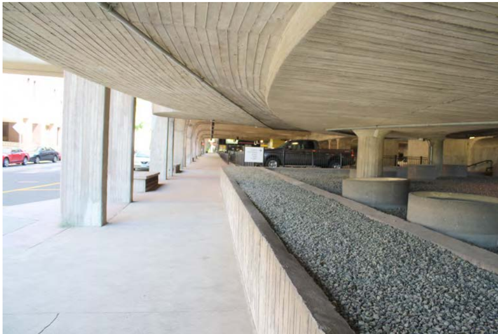
Photo 5. West sidewalk view, camera facing north along Temple Street from Frontage Road. Overhead is the ramp seen in Photo 4 and Figure 22.
