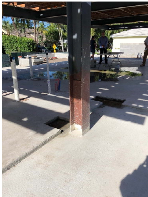
Figure 10. Spliced Steel Column
