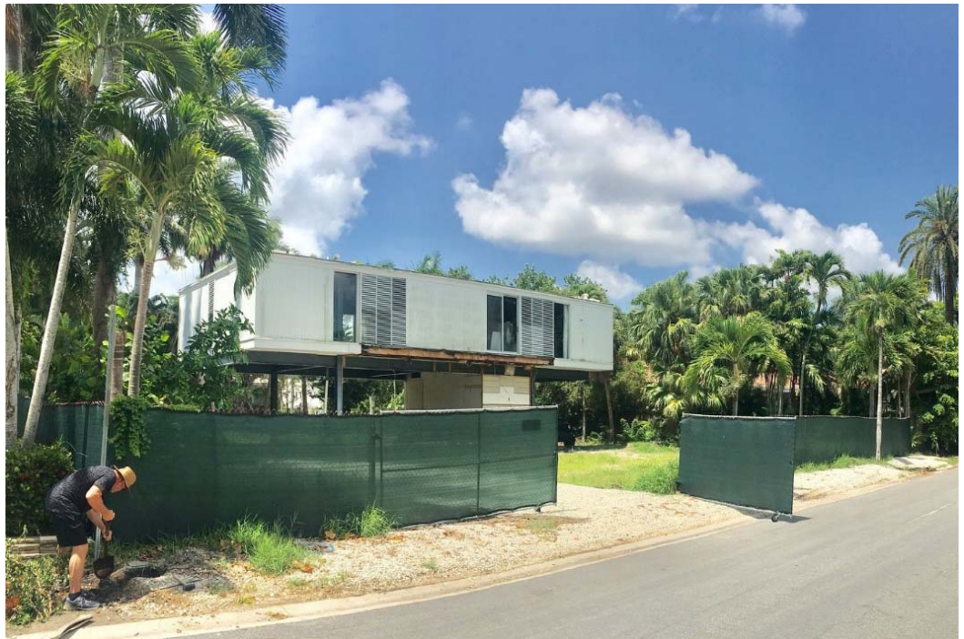
Figure 5. Vista Del Mar South View Following Demolition of additions, 2019
