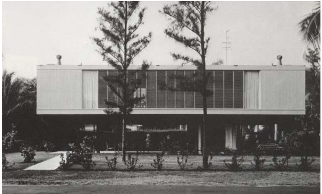
Figure 2. Biggs Residence, Delray Beach, FL – Vista Del Mar Dr. South - Paul Rudolph 1956
