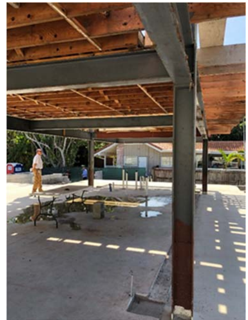
Figure 11. Finish Floor Elevated 18"
