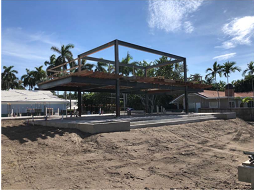
Figure 9. Looking South West from Vista Del Mar South Following Wall Demolition
