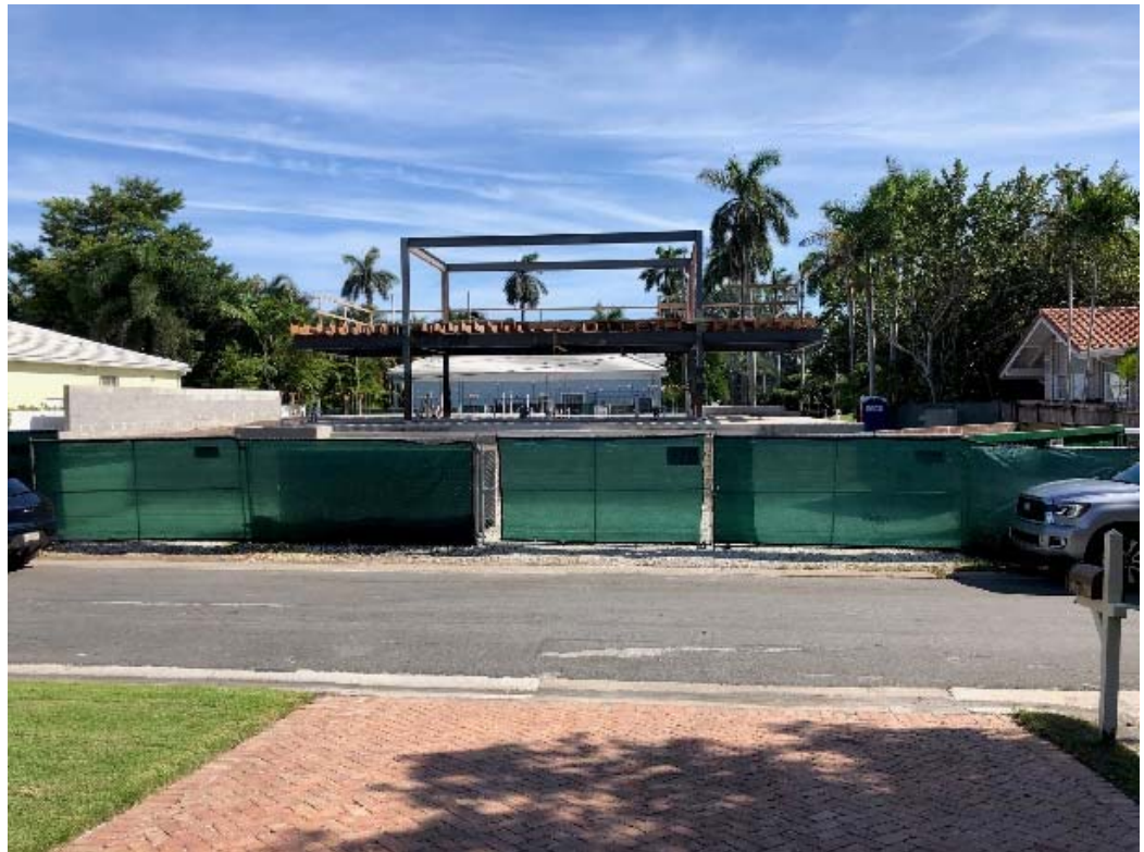
Figure 8. Looking South from Vista Del Mar South Following Roof Demolition
