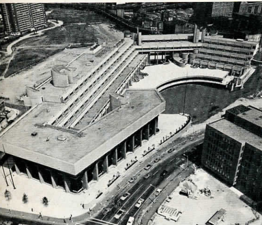
Aerial perspective photo of the State Service Center, tower unbuilt
