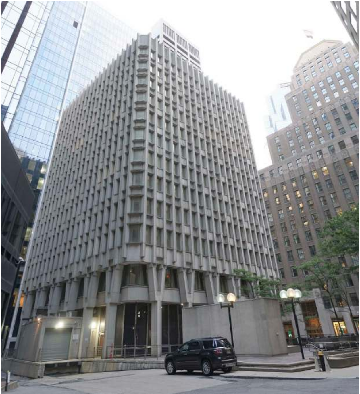
Figure 4. South and east elevations, June 2023. Photo credit: Building Conservation Associates.
