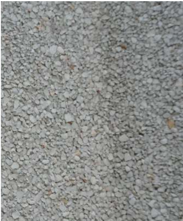
Figure 9. Closeup of Mo-Sai concrete mixture, June 2023. Photo credit: Building Conservation Associates.
