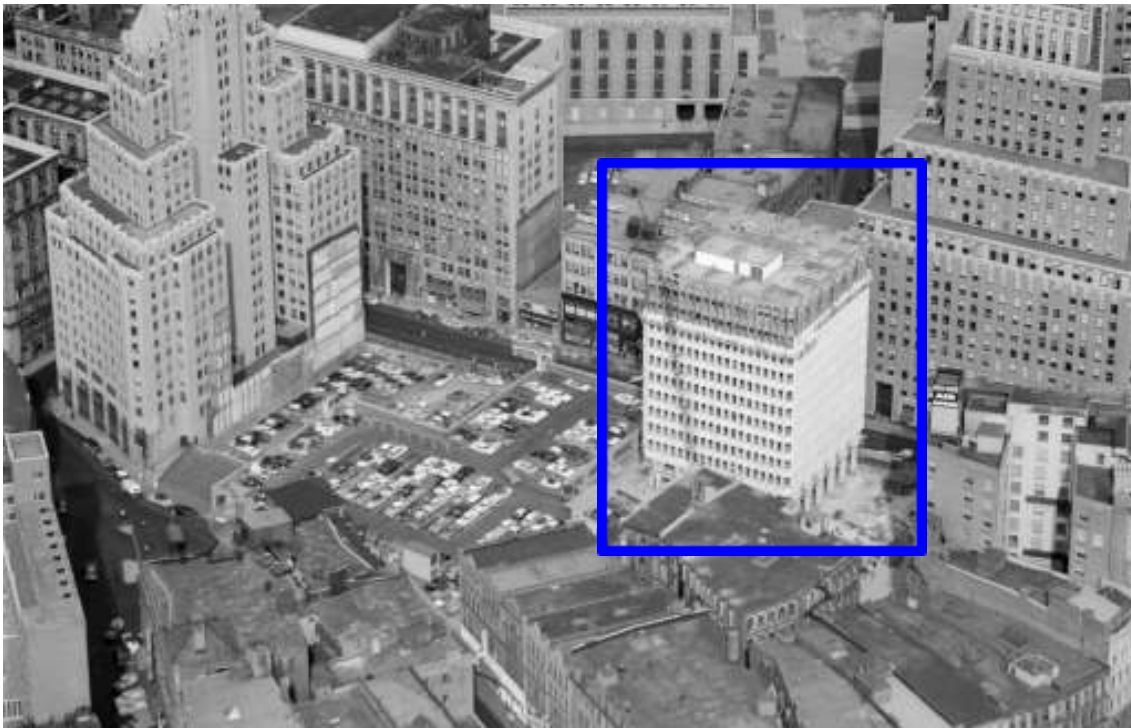
Figure 14. Blue Cross building under construction, Financial District, Boston, MA, 1958-1960.
