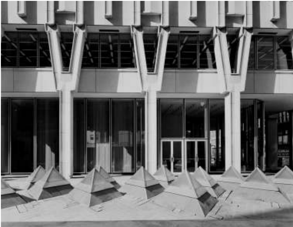
Figure 19. View of exterior plaza showing pyramidal crystalline skylights for the cafeteria below. Photo credit: Joseph Molitor.
