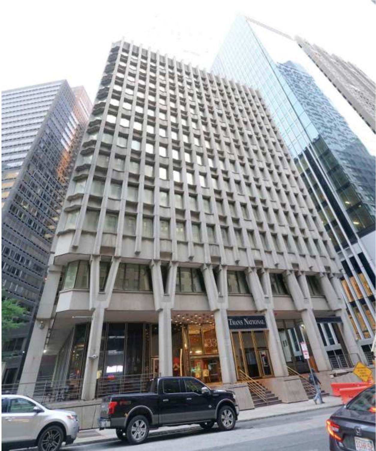
Figure 2. East elevation, June 2023. Photo credit: Building Conservation Associates.
