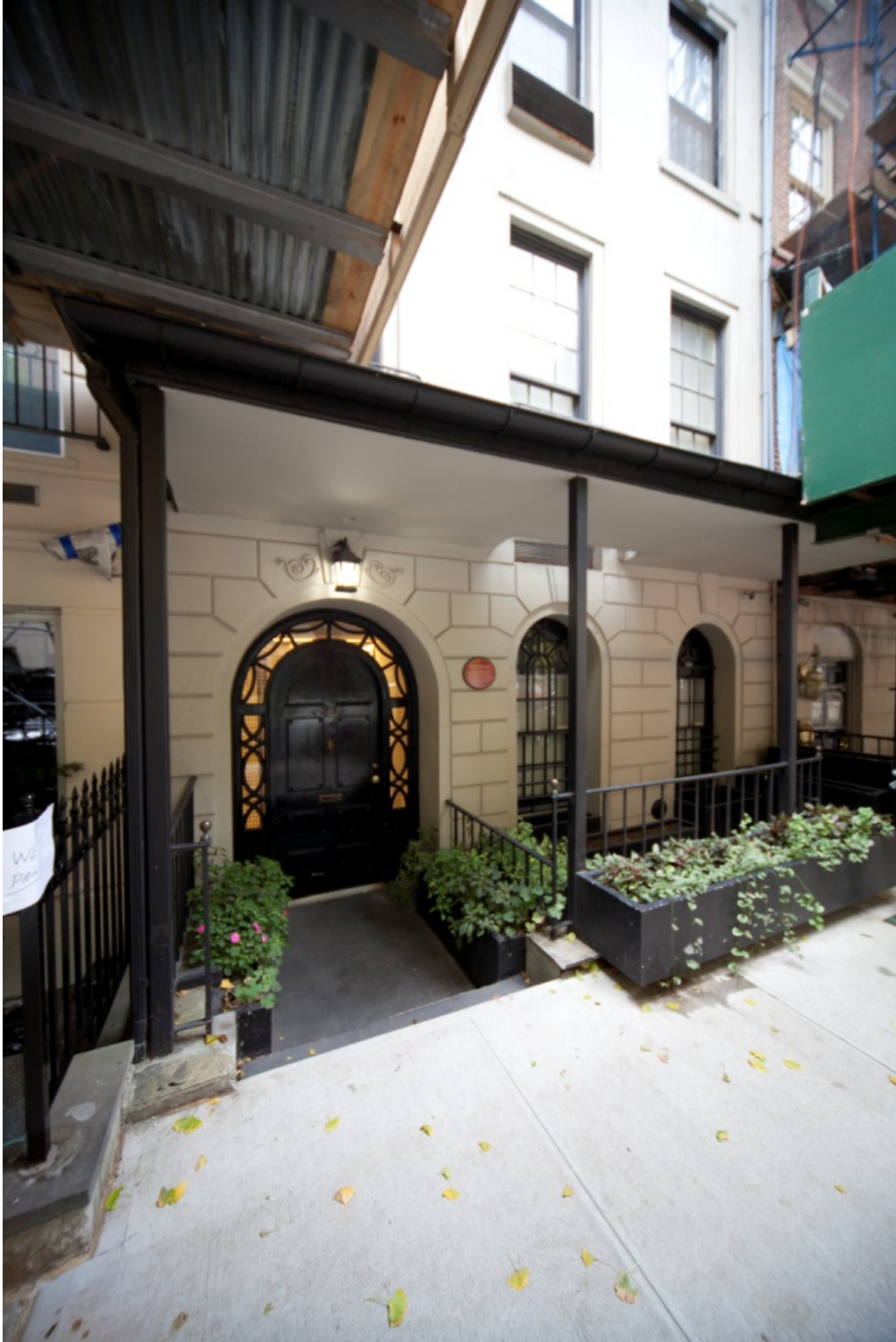
Paul Rudolph Penthouse & Apartments Beekman Place, entrance Photo: Christopher D. Brazee, 2010
